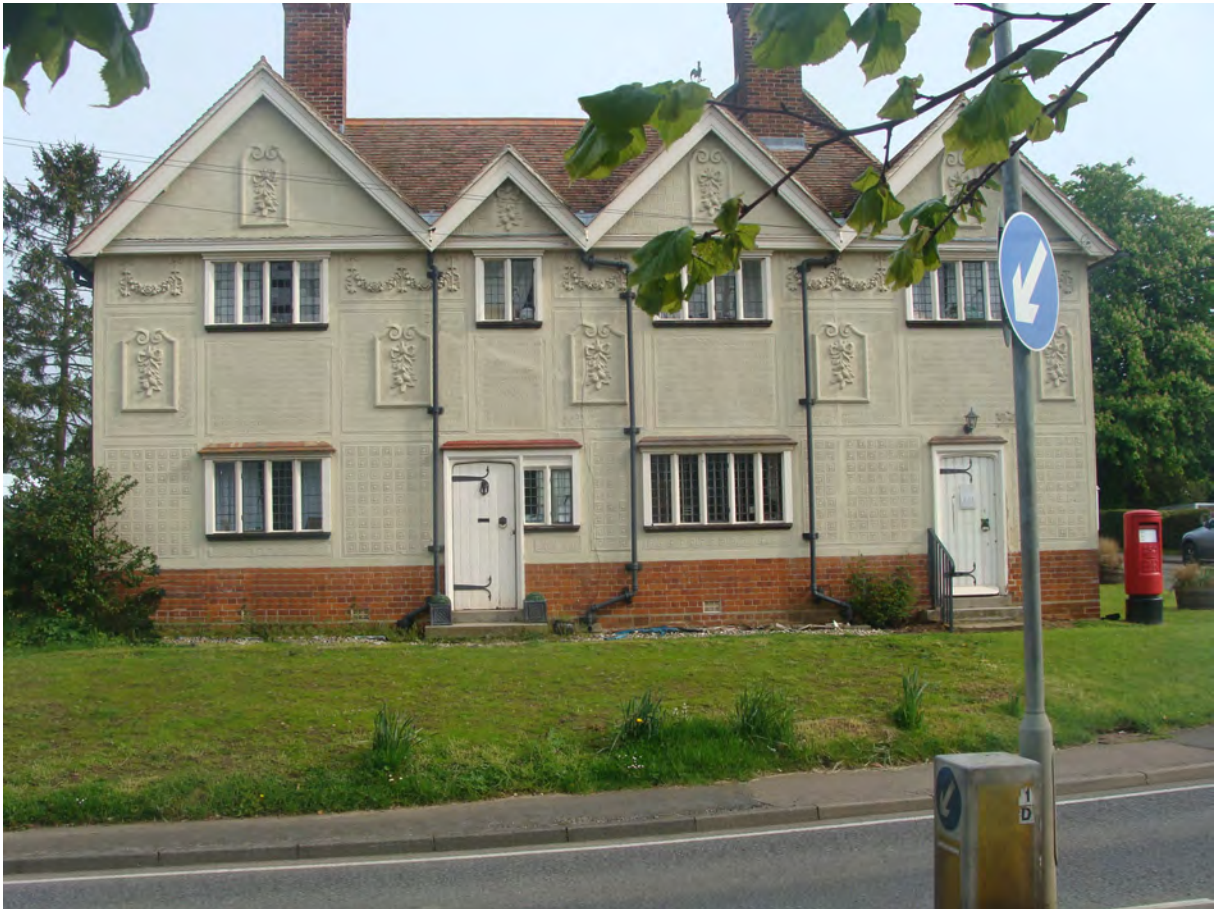
Picture 1.13 Now the Parish Hall and cottage, formerly a Reading Room and Dispensary
