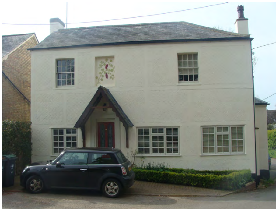
Picture 1.3 The building today, original commercial window detailing replaced and large central porch added. Change of use may have been inevitable but a more appropriate design solution retaining some original features would have been possible
